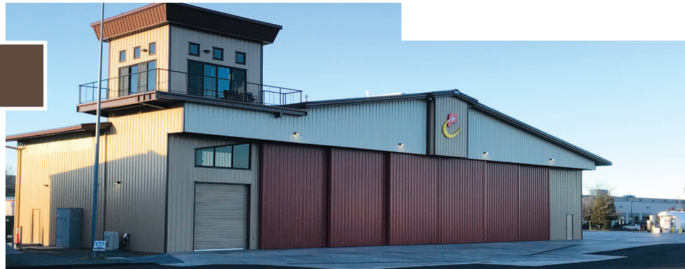
PROJECT: FLYERS ENERGY HANGAR
